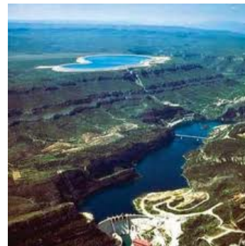
LaMuela, Spain (635 MW)
